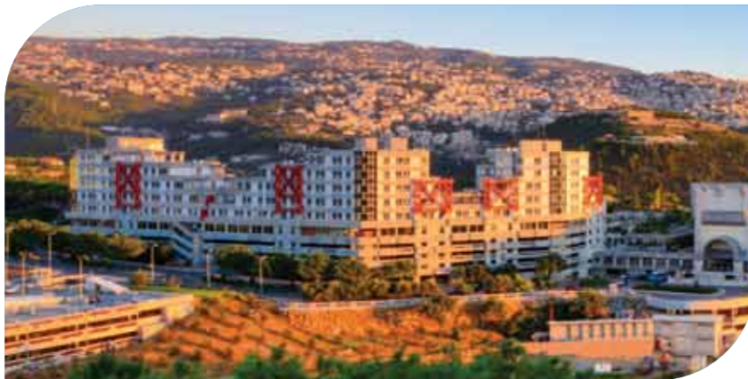
A view from the top: Fr. Bechara Khoury oversees construction work from a crane on the Main Campus.
